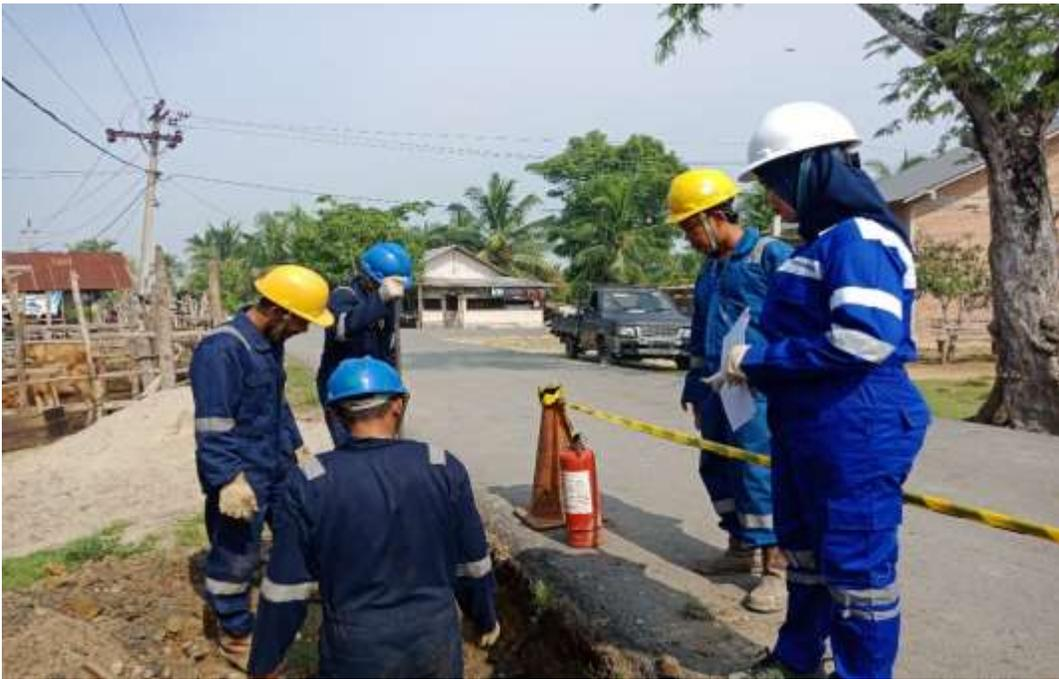
**Gambar 2. Proses Pencarian Kebocoran Pipa Gas**
