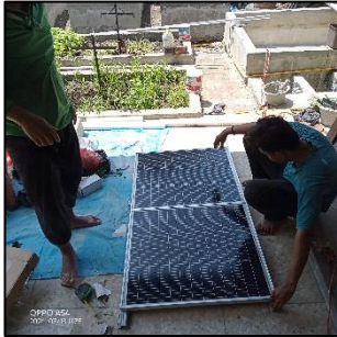
3. Pengecekan tegangan panel surya
