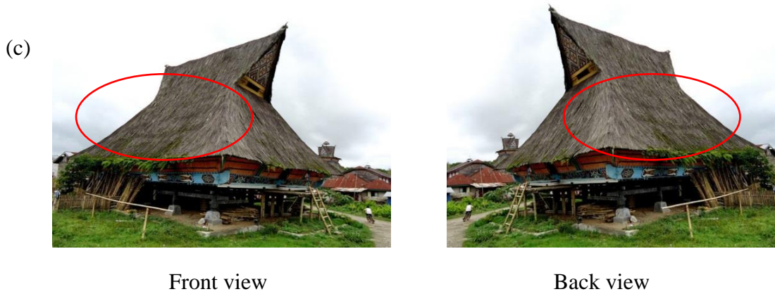
Figure 8. Roof of Karo Traditional House
