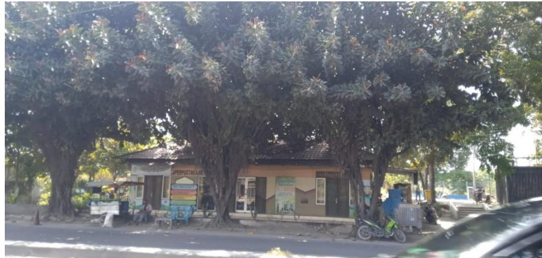
(Gambar 1. TBM Tampak Depan)
