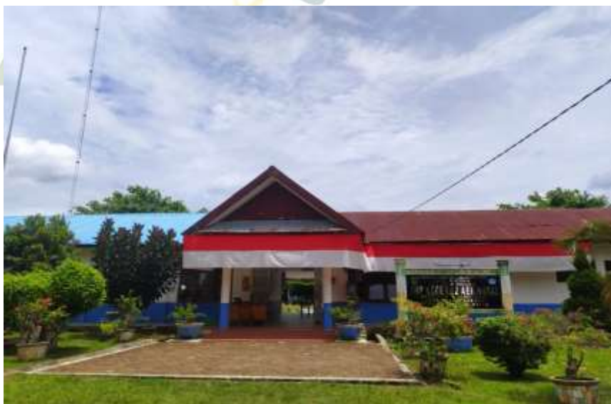
School building of SMPN 2 Aek Natas
