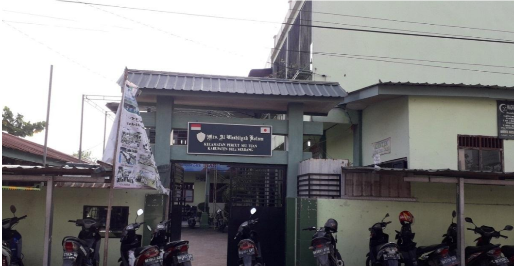
Gerbang MTs Al-Washliyah Kolan
